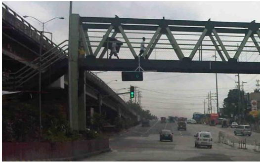
Figure 1: A truss used in a footbridge
